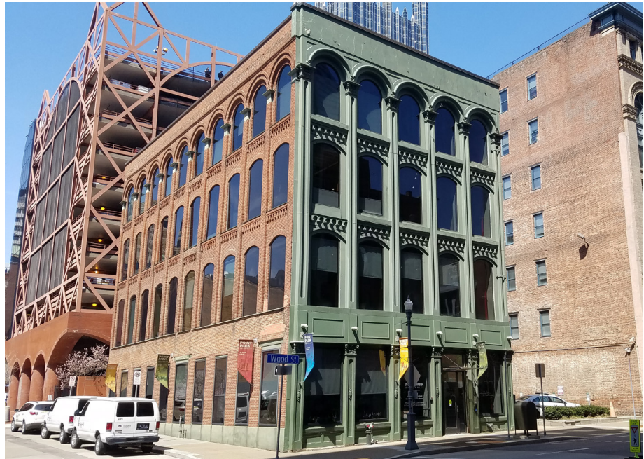
101 Wood Street - location of the new Welcome Center and proposed Admissions Center
