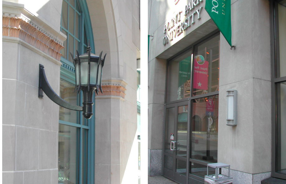
Examples of Existing Sconces on University Buildings
