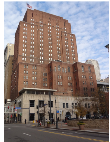
improvements to the lower level facades)
